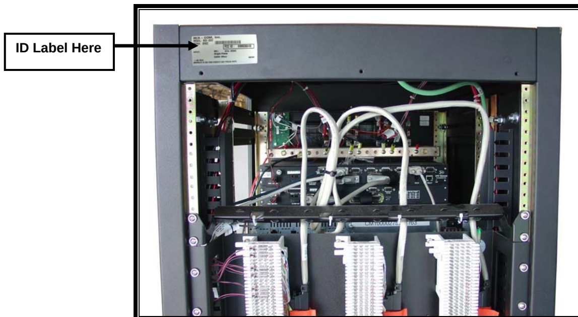
Photograph 2: ID Label Location
