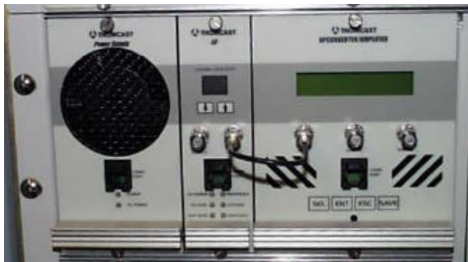
Figure 1: Cabling the LO signal.
