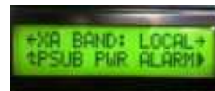
Example of system status with active alarms
