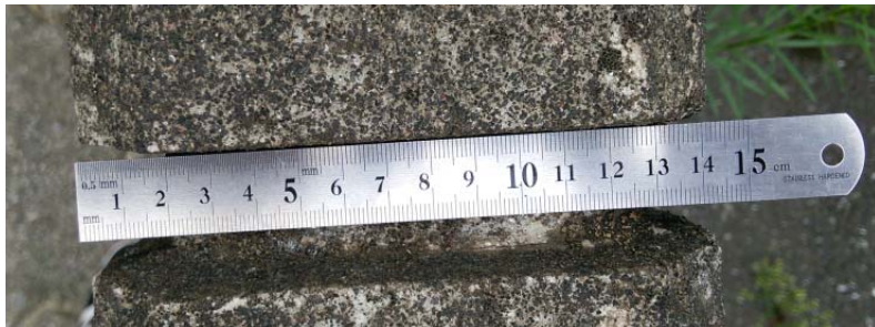
Figure 6-1 Confirmation of the wall width
