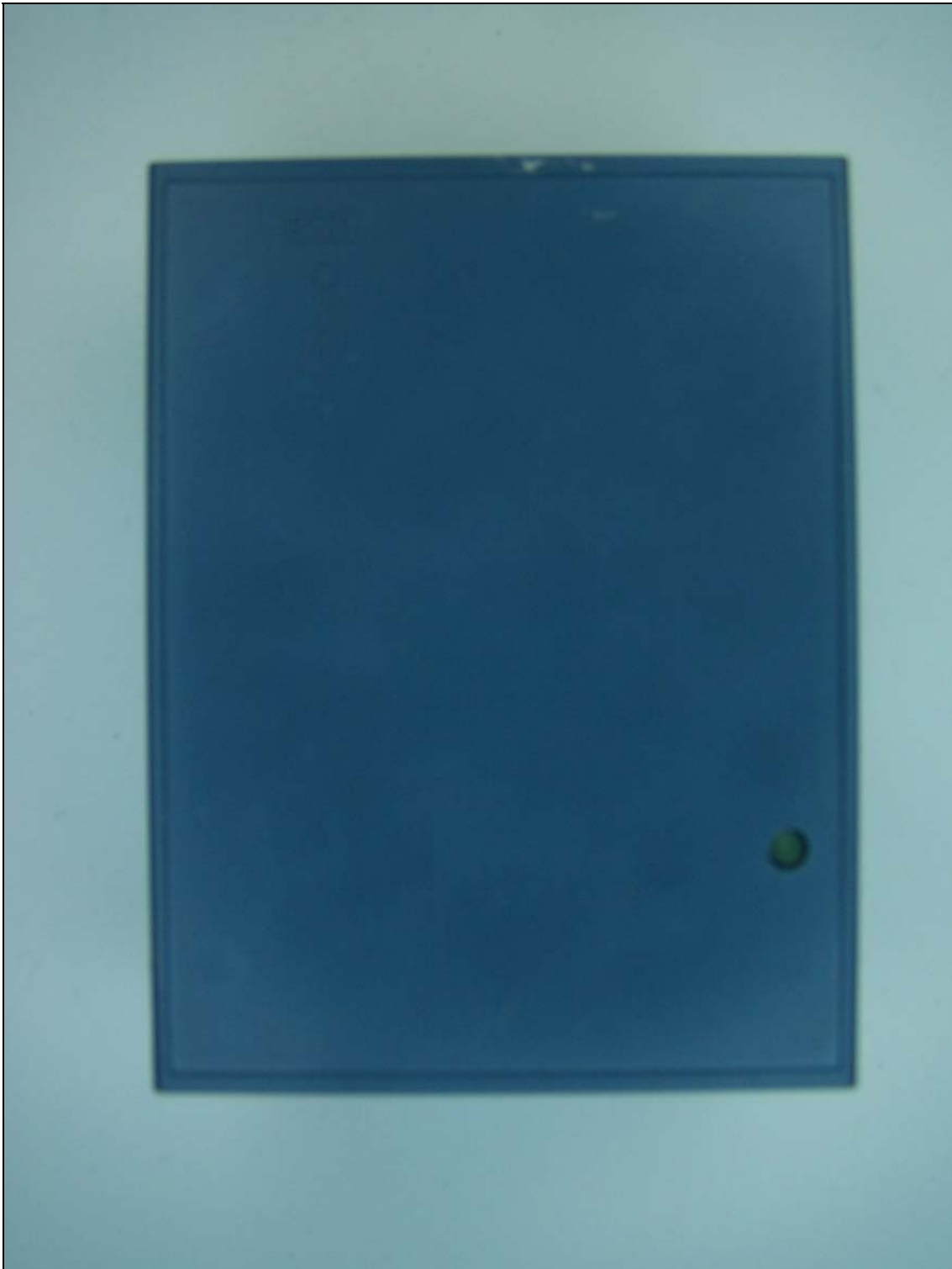
Photograph 10. External Photograph, Front View
