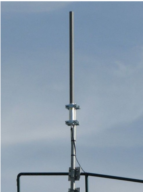
Remote 8.15 dBi 915 MHz antenna: 68.0" L x 2.0" D
