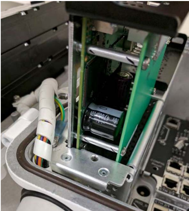
Figure 84 Sliding the Existing CAM Out of the CGR
