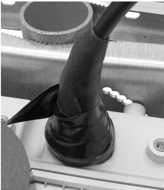
Figure 37 Electrical Tape Application Around the Butyl Rubber
