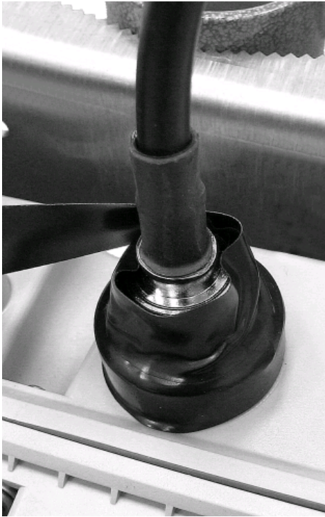
Figure 34 Starting the Electrical Tape Application
