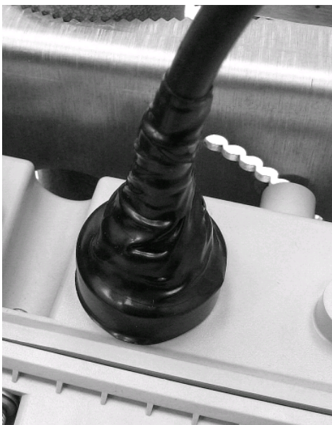
Figure 35 Fully Covered Electrical Tape Application
