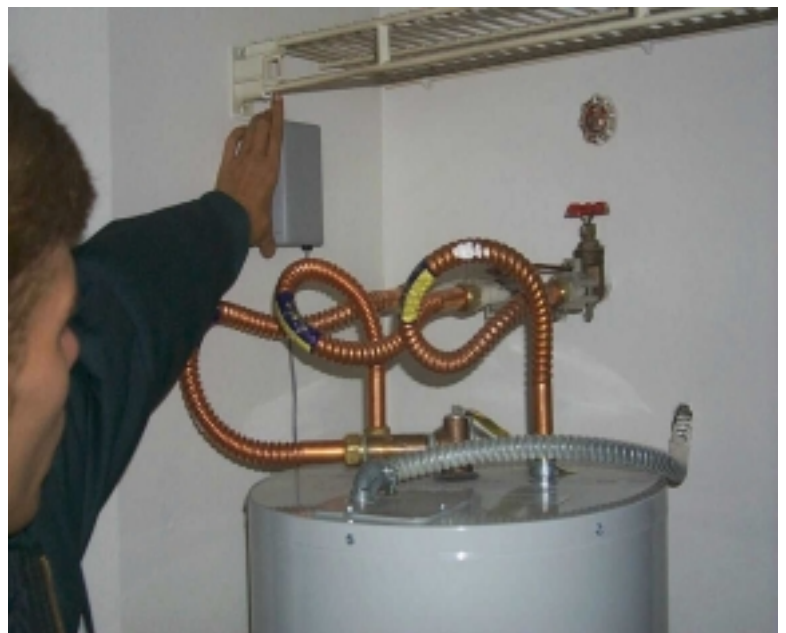
Water Meter with Transducer
