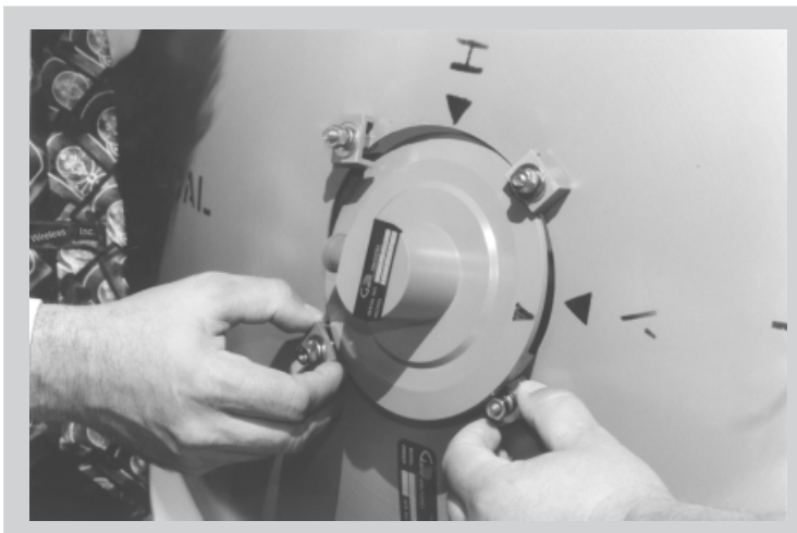
Figure B.13 - Feed Horn Installation
