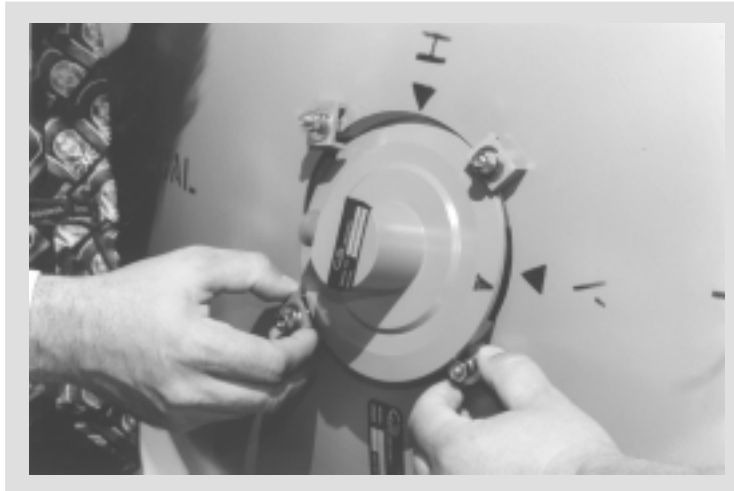
Figure B.13 - Feed Horn Installation
