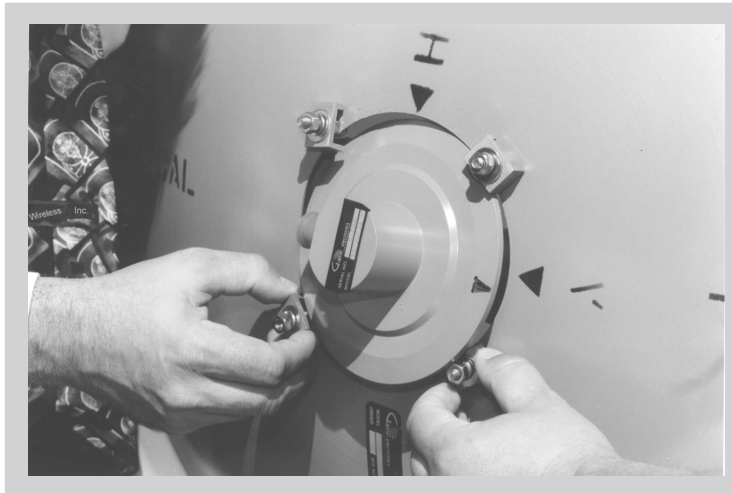
Figure B.13 - Feed Horn Installation
