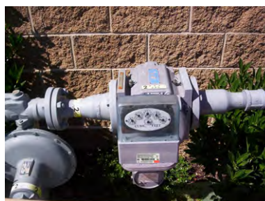
Sensus commercial 500G ERT module mounted on a GE Oil and Gas meter with an instrument drive
