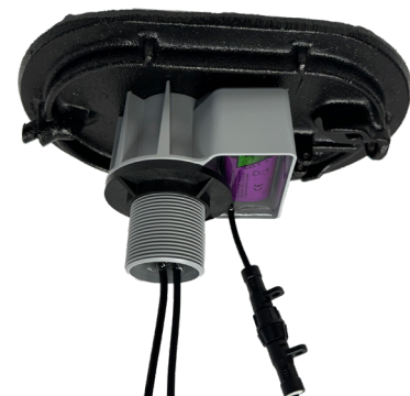
Figure 8: View from under pit lid
