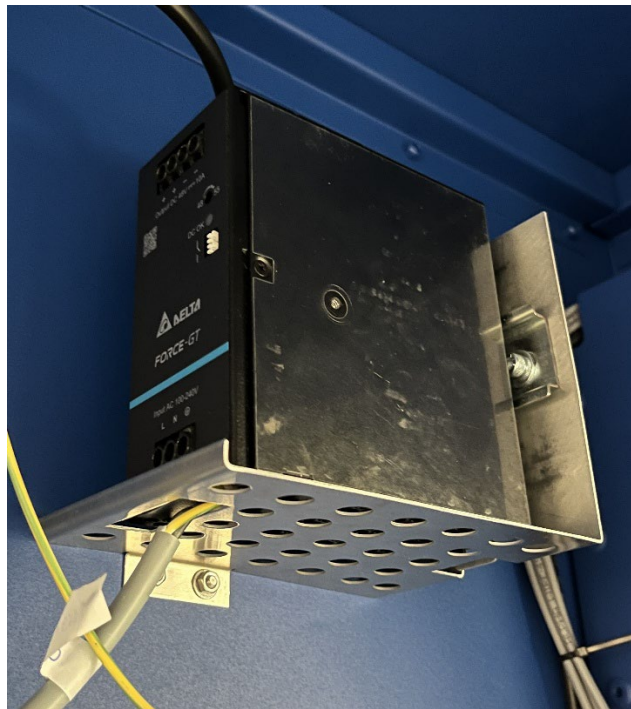
Power supply unit, oblique view
