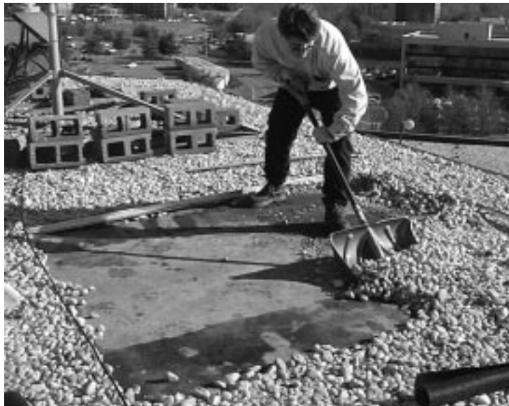
Figure 5-2 Clearing gravel from the installation location
