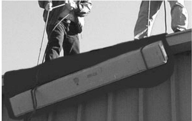
Figure 4-1 Hoisting materials to the installation location
