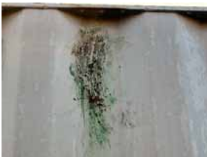
Figure -4 Dirty, greasy mount location
