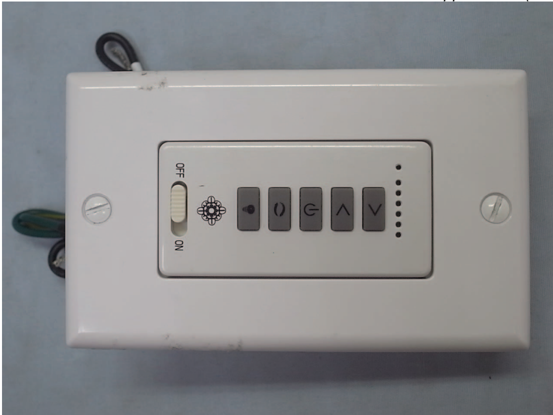
Photo 1 General Appearance (Front View)
