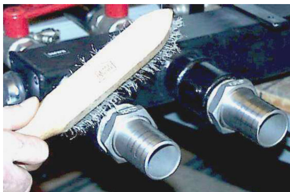
Figure 4-44: Removing protruding hemp frays.
