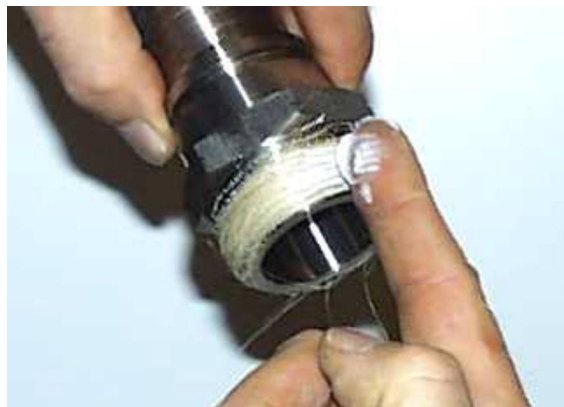
Figure 4-42: Coating thread with sealant.
