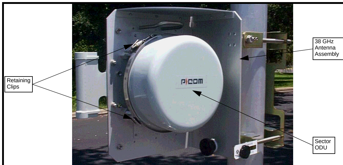
Figure 6-8 - Attaching 38 GHz ODU to Antenna Mount Assembly
