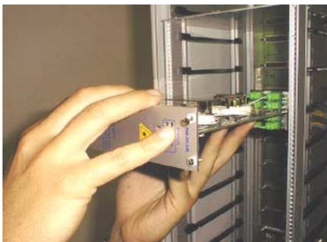
Figure 12 Installing the LU
