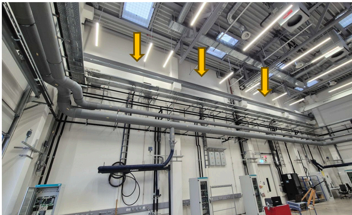
Photo 2: Installation of RCoax x cable in the test location; the yellow arrows point to place where the RCoax cable is installed
