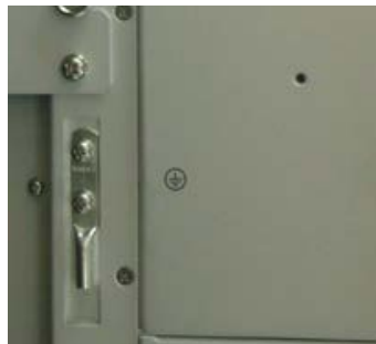
Figure 4-2 Ground Cable Connection
