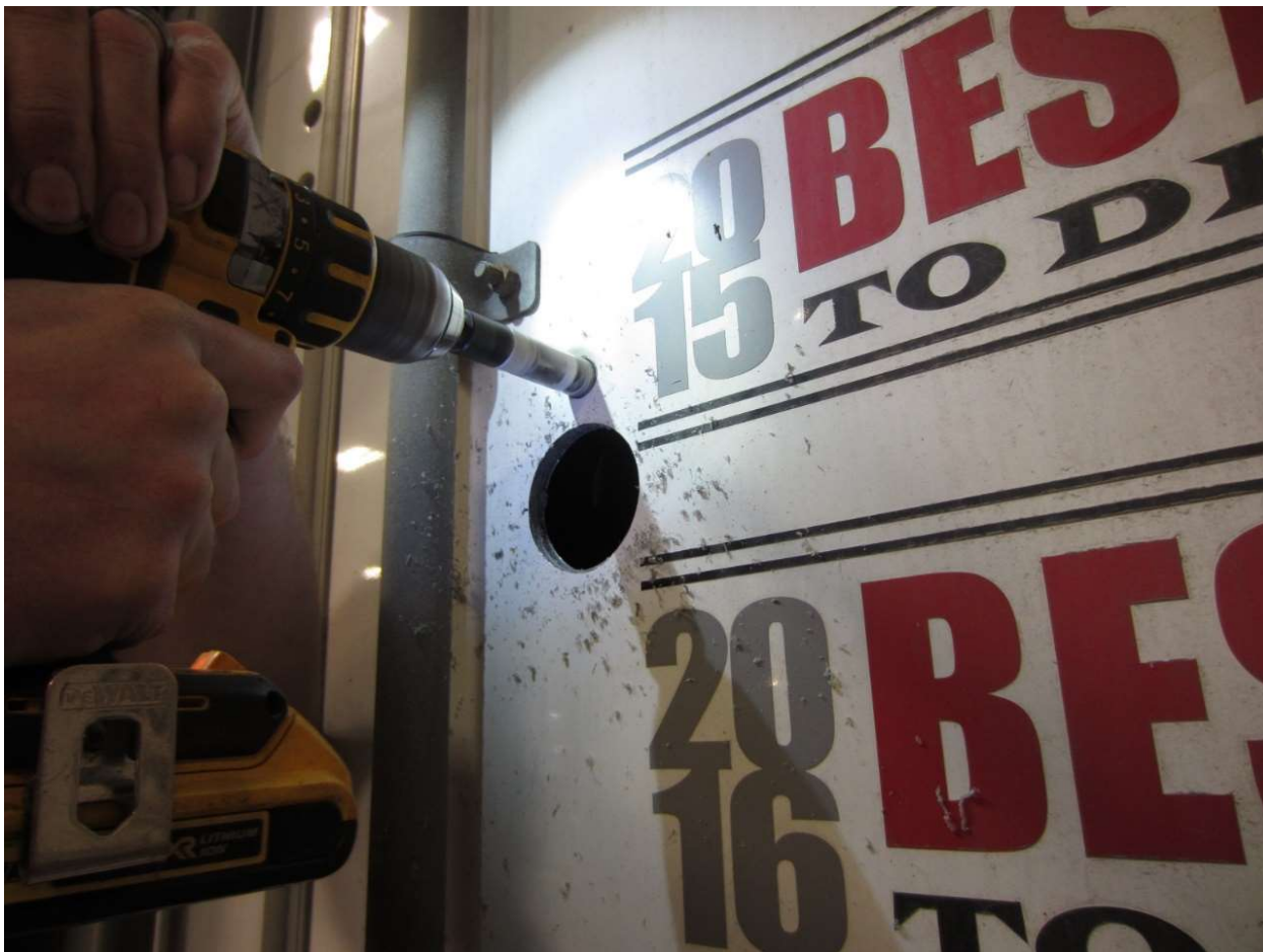
\frac{3}{4} " hole for positioning dowel
