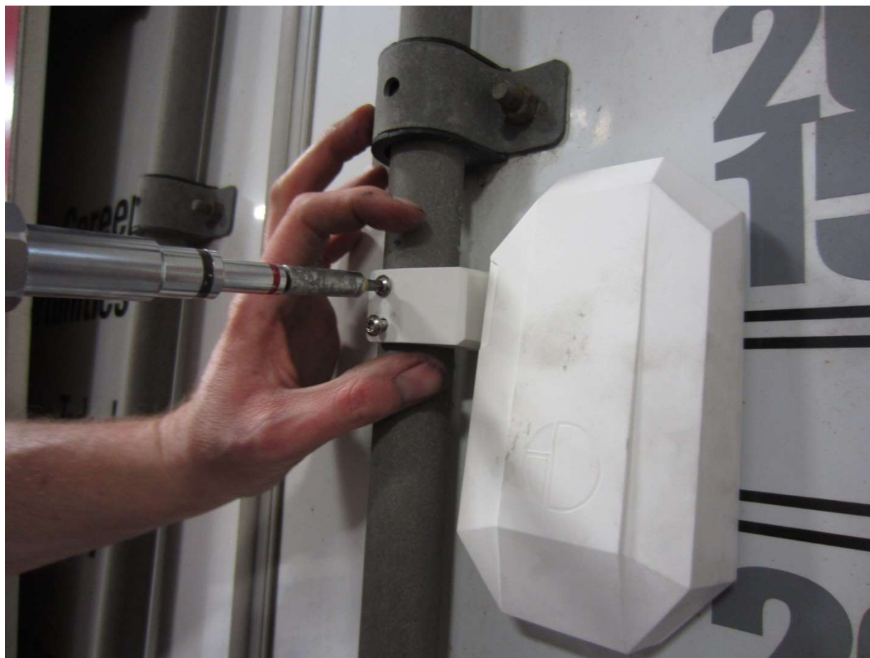
Install thread forming screws
