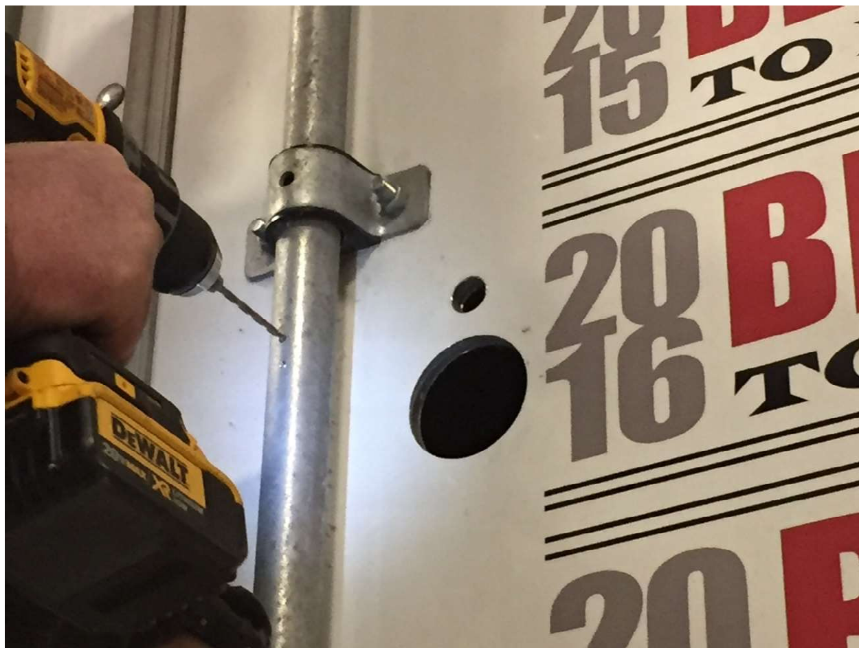
Drill #17 holes in inner locking rod
