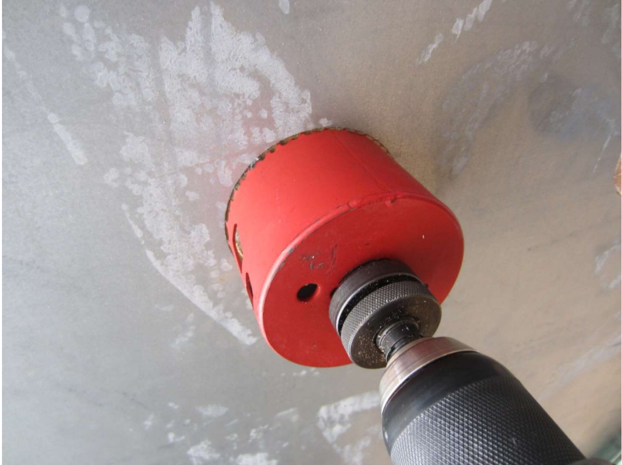
Drill 3 3/8" hole through interior door sheathing
