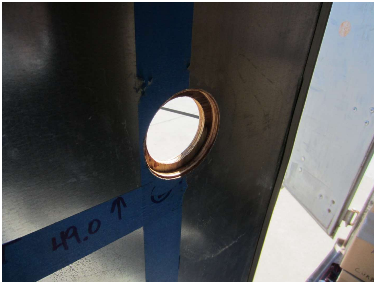
Countersink around lens hole
