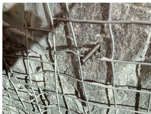
Plate Step 3. Insert both Anchors
