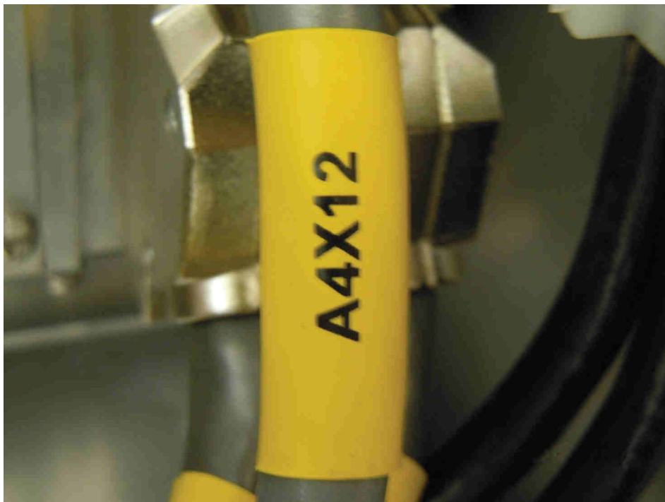
Fig. 7.10 Marking, other cables
