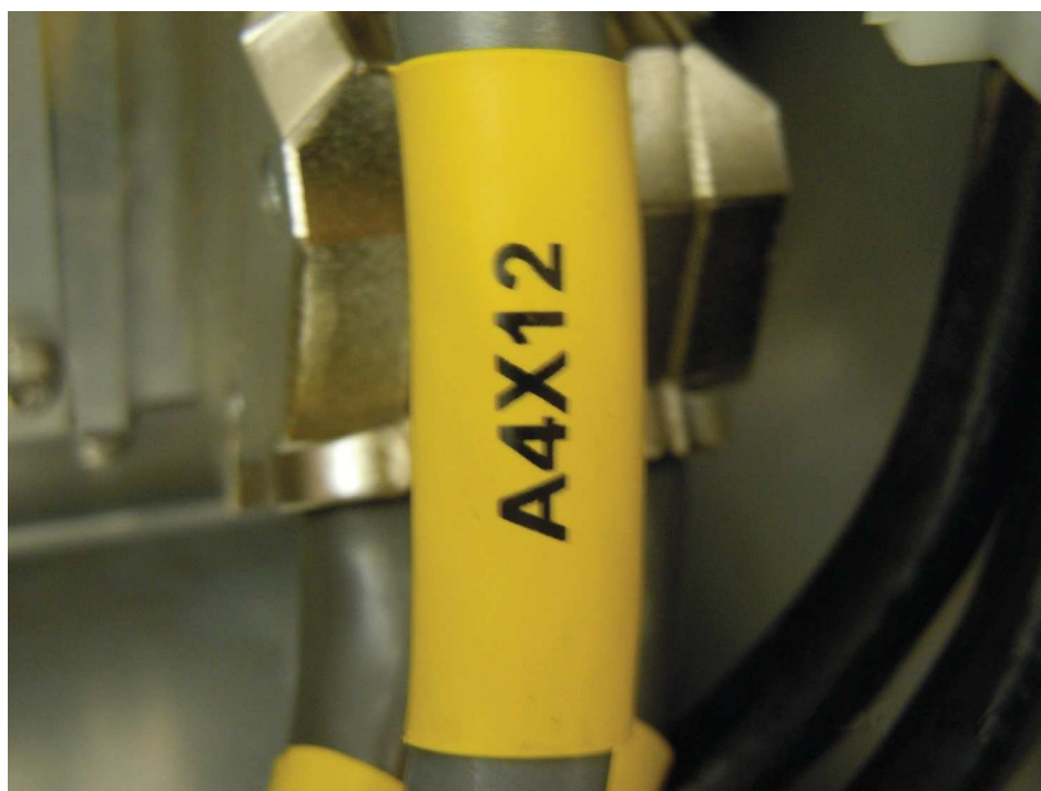
Fig. 7.4 Marking, other cables
