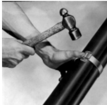
Fig. 3.14. Hammering buckle ears
