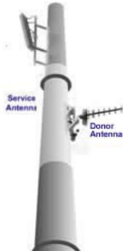
Figure 2-3. Service above Donor Antenna
