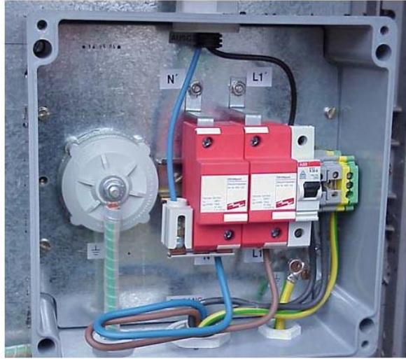
Figure 3-24: Protective device installed in connection with the power supply
