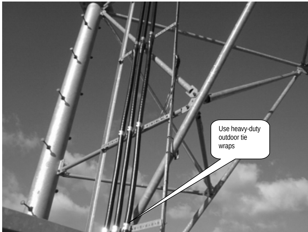
Figure 2-3. Fasten IF Cables to the Tower
