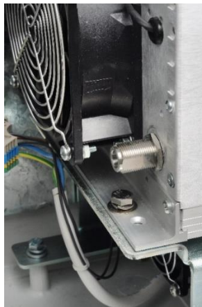
Bolt Securing Base Station to Cabinet
