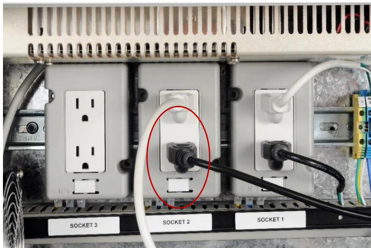
Connect Power Cables to Cabinet
