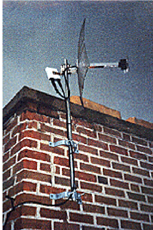
Figure 3-2 High Gain Reflector Antenna Installation
