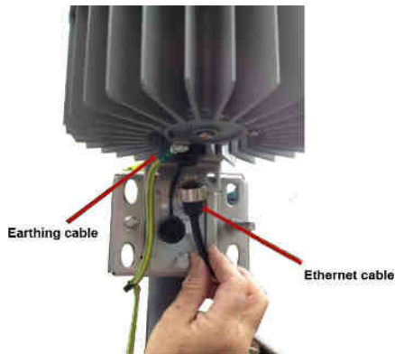
Figure 25: iR460 with Earth and Ethernet Cables Installed
