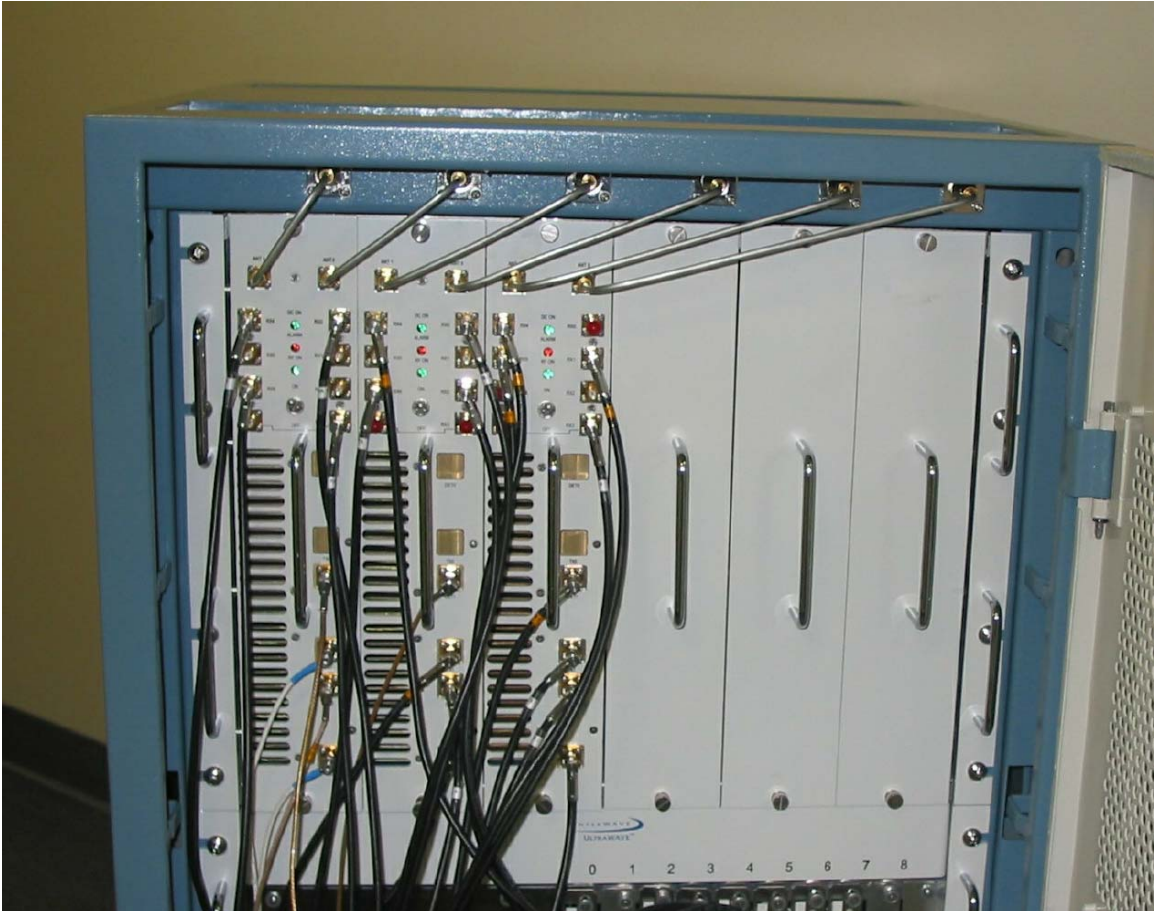
RF-Module in Base Station UltraWAVE BTS, AUAC85
