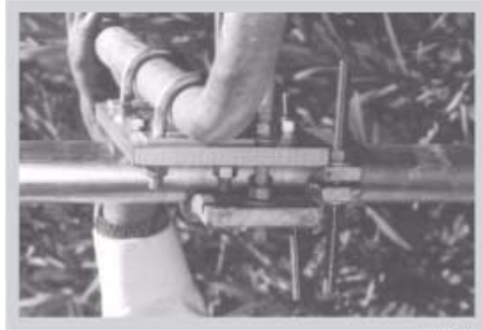
Figure 4-29 Azimuth Adjustment Clamp Assembly
