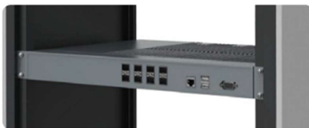
Figure 8. Place A2 in Rack
