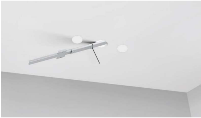
Figure 64. Placing the Bracket I & VI
