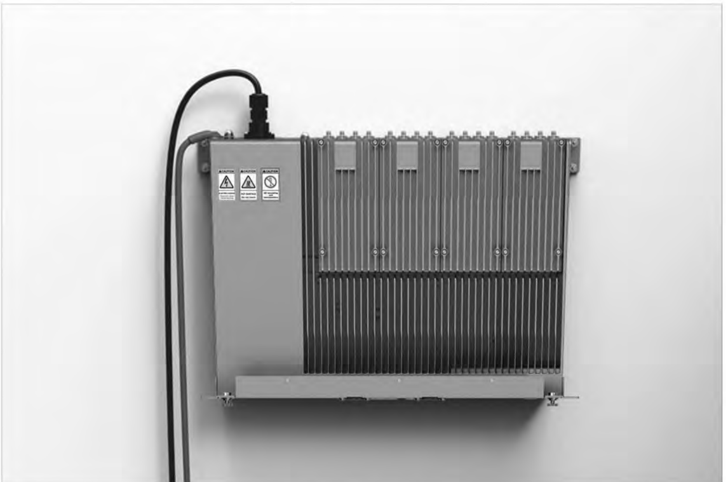
Figure 13. A3 Wall Mounting Completed
