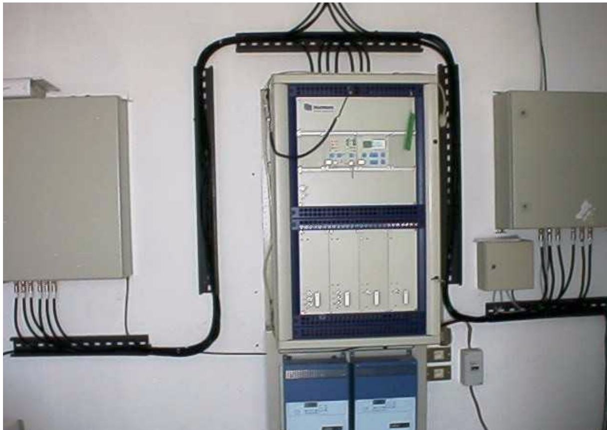
Figure1-4 Localizer Cabinet Installation
