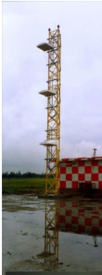
Figure1-3 Glidepath Antenna
