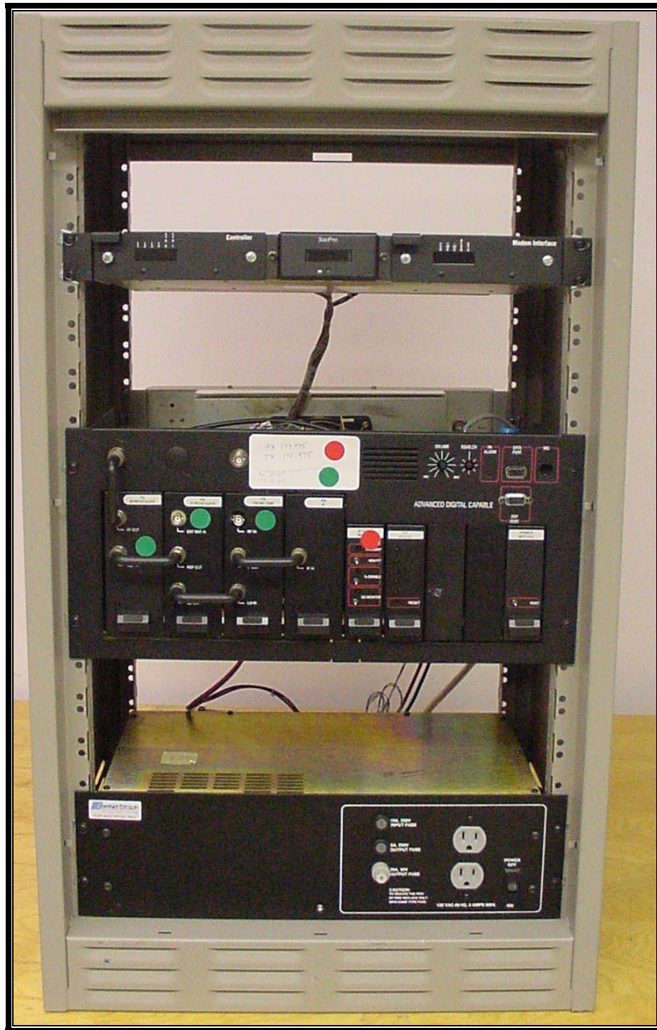
PHOTOGRAPH 3: MASTRIII FRONT VIEW
