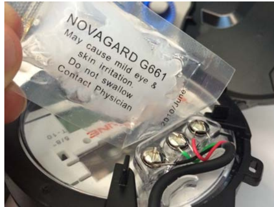
Figure 5 Application of the Sealant
