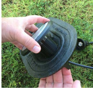
Figure 28 – Inserting the Antenna into the Pit Lid
