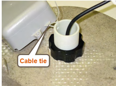
Figure 31 – L900 MIU Attached to Antenna
