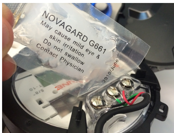
Figure 11 – Application of the Sealant
