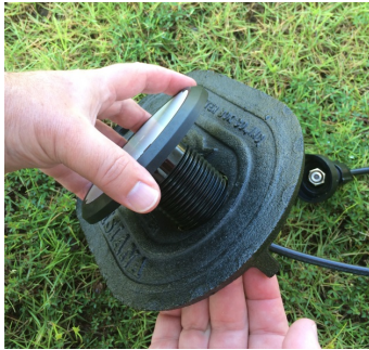
Figure 26 – Inserting the Antenna into the Pit Lid
