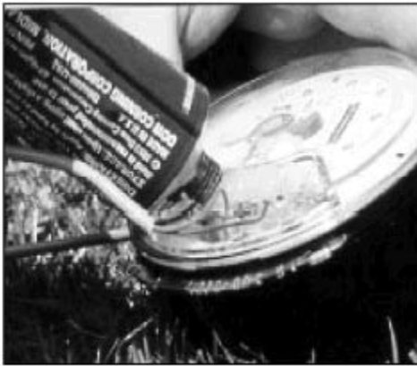
Figure 2.6 Installing Moisture Protection Compound
