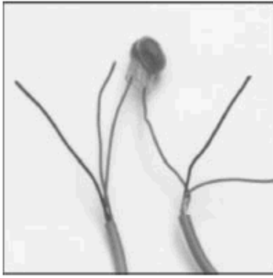
Figure 2.13 Unstripped Wires in a Scotchlok
