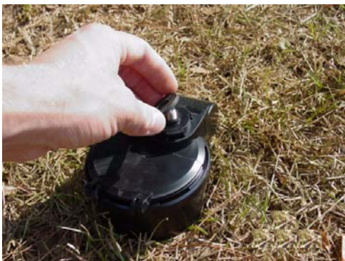
Figure 15 Placing Washer on MIU
