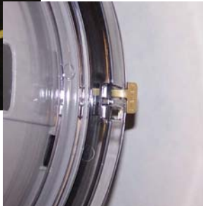
Figure 10 – T-Seal Installed
