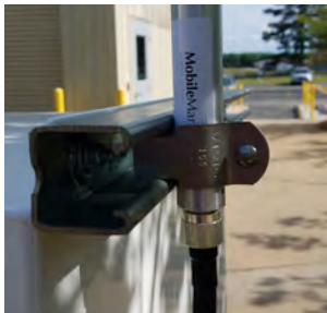
Figure 11 – Attaching the Cellular Antenna
