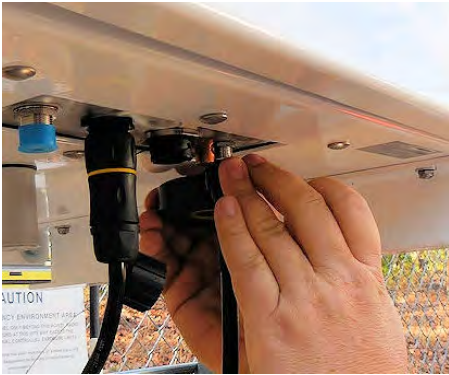
Figure 16 – Weatherizing the Base Connection
