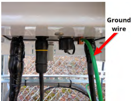
Figure 9 – Ground Wire
