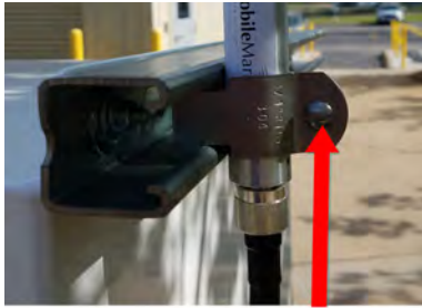
Strut clamp bolt
