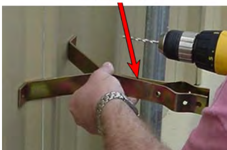
Figure 54 – Securing the Pole Bracket
