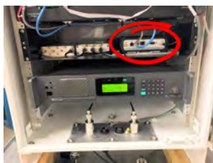
Figure 27 – Modem in R450 RMDC
