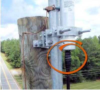
Figure 57 – Weatherizing the RF Antenna Connection
